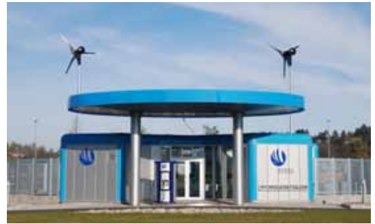
Hydrogen station, Statoil (former StatoilHydro)
